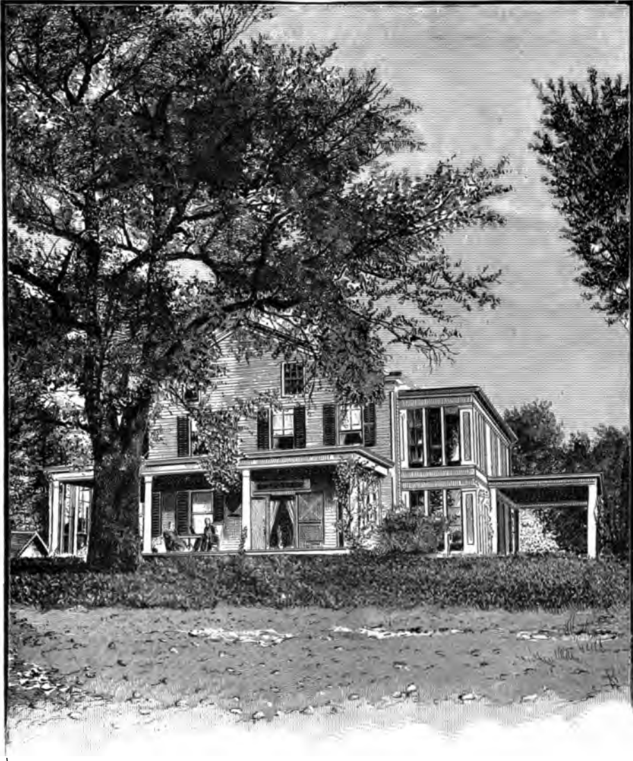
HOME OF HORATIO SEYMOUR AT DEERFIELD. FRONT OF HOUSE, SHOWING THE BROAD PORCH. [Engraved from a Photograph.]
